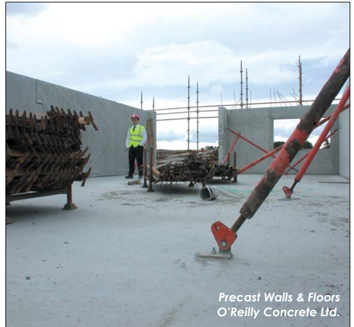
Adamstown Apartments, Dublin O'Reilly Concrete Ltd.
