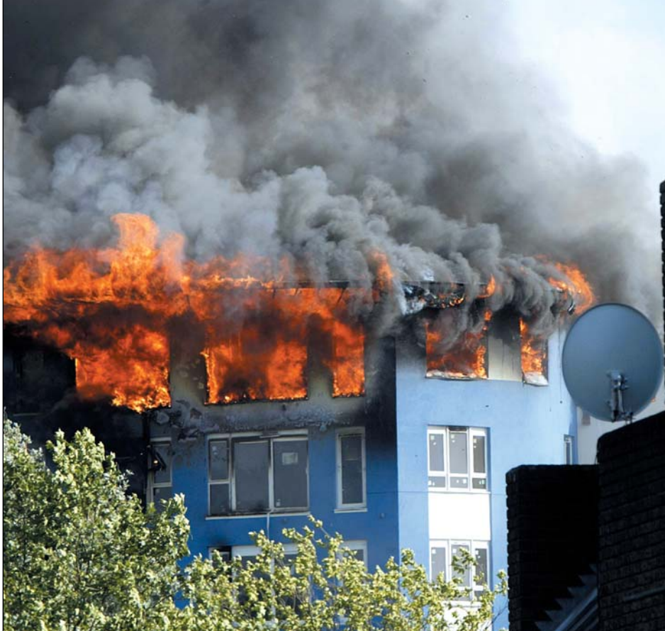
Timber frame fire – Colindale, London
