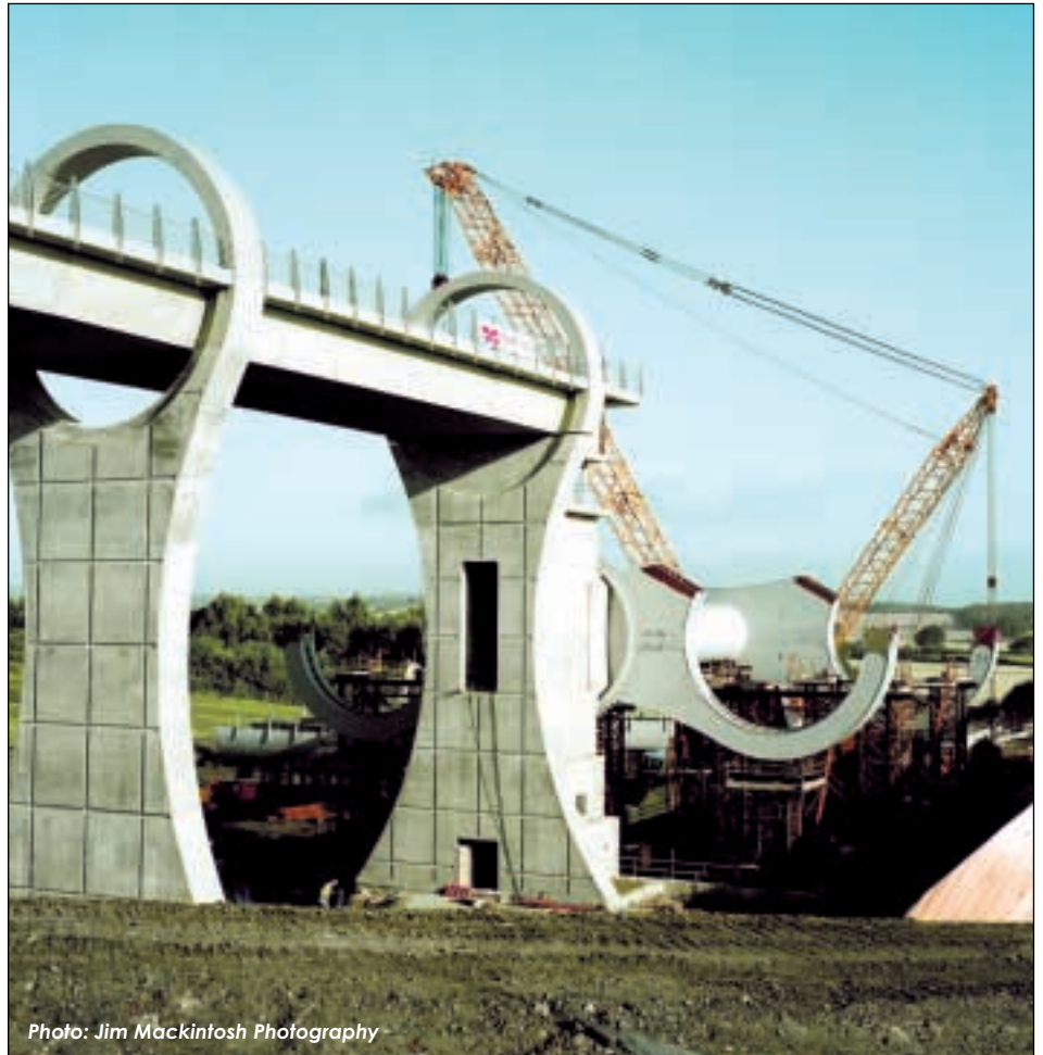
Figure 2: Erection of the wheel after completion of the concrete structure.
