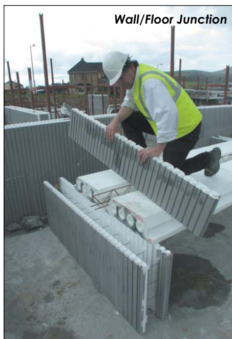
Typical Wall Assembly
