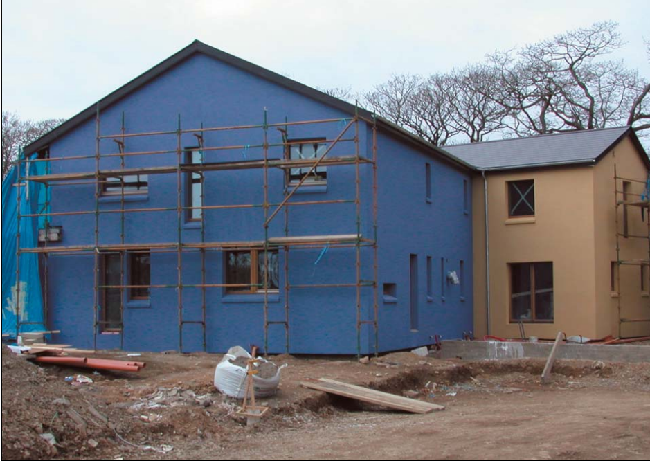
EPS insulation rendered with acrylic plaster
