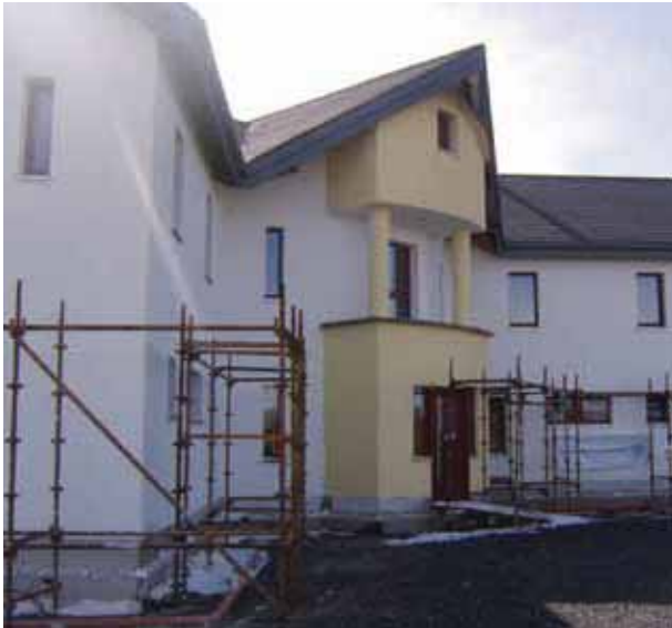
The ICF supported Zero Carbon Emissions House under construction.
