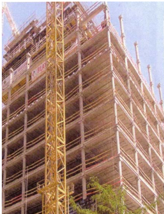
Figure 1.3: The North Galaxy Towers in Brussels. This reinforced concrete 30-storey concrete building meets the current strict requirements for fire resistance (REI 120); the columns are of high-strength C80/95 concrete. (Courtesy ERGON, Belgium)
