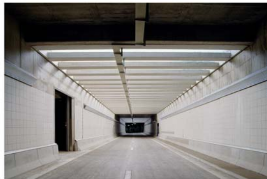
© photo-daylight.com. Copyright free for all publications edited by CEMBUREAU/BIMERMCO Members including web sites Kinkempois Tunnel (link E25-E40) in Liege, Belgium, using concrete pavement
