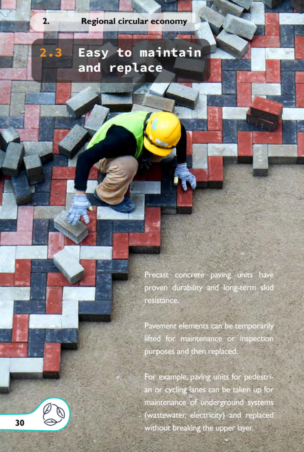
Precast concrete paving units have proven durability and long-term skid resistance.
